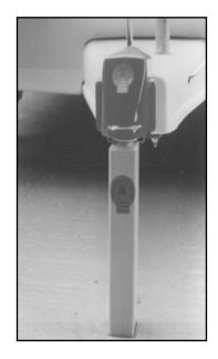
3. When the concrete is set, hitch up your caravan or trailer to the post and lock on your Bulldog Minilock.
